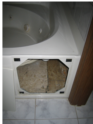
Missing whirlpool motor
