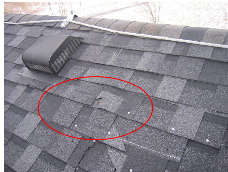
2nd area of repair to roof
