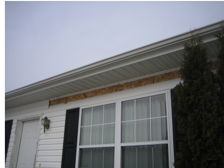
Repair siding south face
